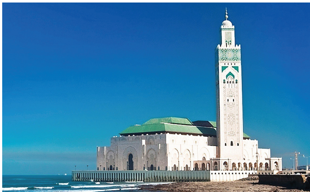
Fig. 6. Hassan II Mosque, Casablanca, Morocco. 1986–1993.
