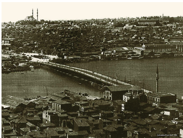
Fig. 3. Unkapanı bridge built over the Golden Horn
