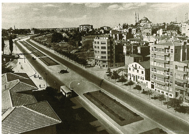
Fig. 4. Atatürk Boulevard view from Aksaray
