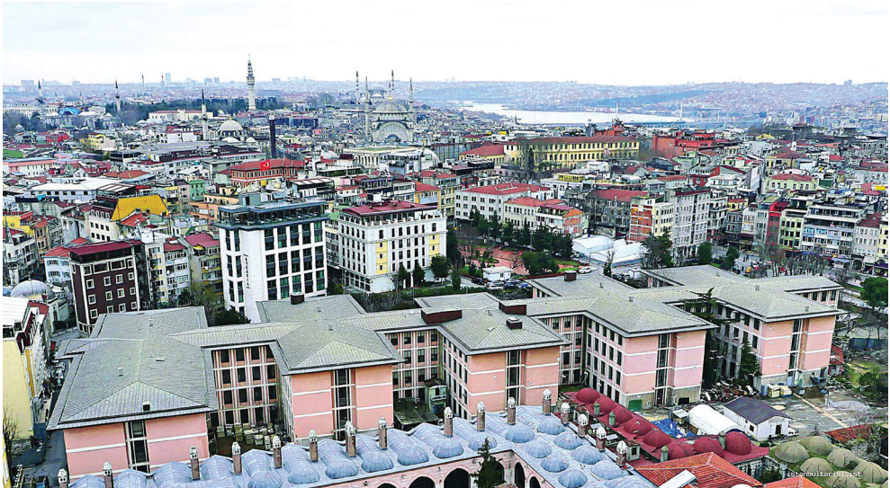
Fig. 12. Sultanahmet courthouse building
