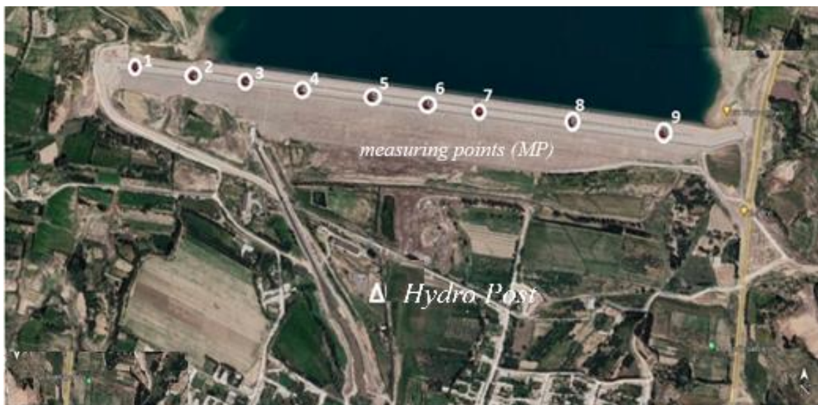
Figure. 2. Location of registration points in the dam body Chartak Reservoir
